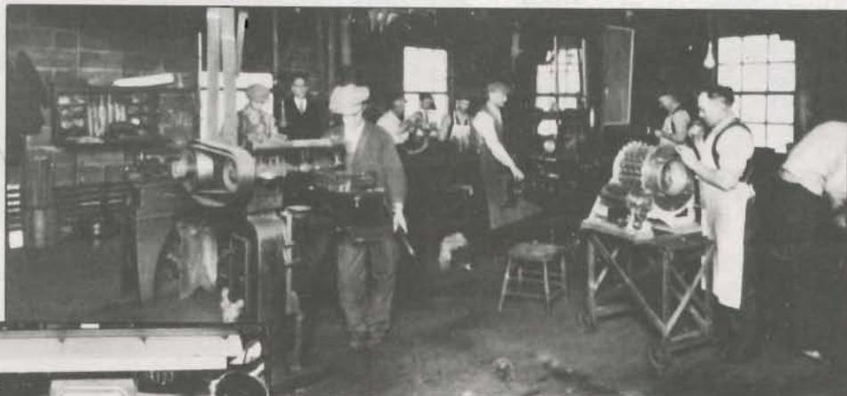
About 1929 at the plant on South Napoleon Street – The machine shop was located in a number of small rooms. All the machine tools in each room were driven by a single large motor through line shafts and belts. William Urschel (left background) supervises the operation.
