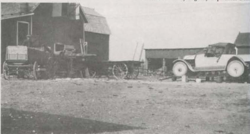
Homemade car being used to power corn shredder
